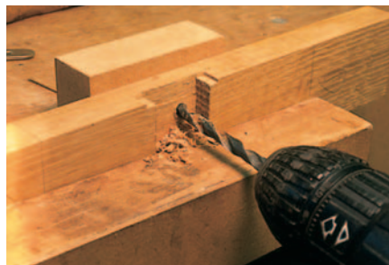
Fitting lock. Drill hole for pin, just bigger than diameter of key barrel
